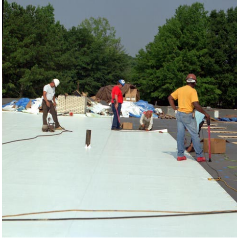
White Roof of Commercial Building
