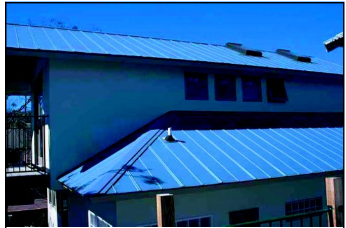
Metal roofs can last decades longer than asphalt shingles
